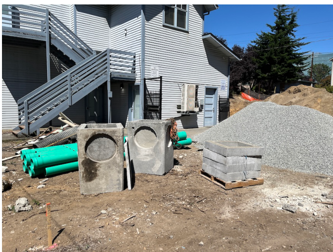
Stormwater drainage components for the parking lot. The one in the right photo is shown in place, and will feed into the detention vault. (July 16)
