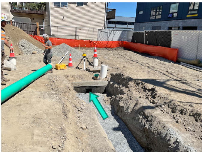
The green pipe goes into the hole in the side of the detention vault. (July 16)
