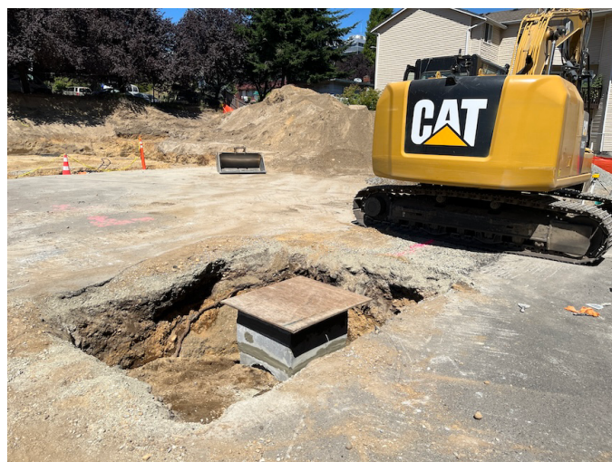
Stormwater drainage components for the parking lot. The one in the right photo is shown in place, and will feed into the detention vault. (July 16)
