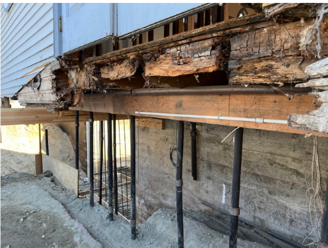
A good view of the deterioration below the old lobby
